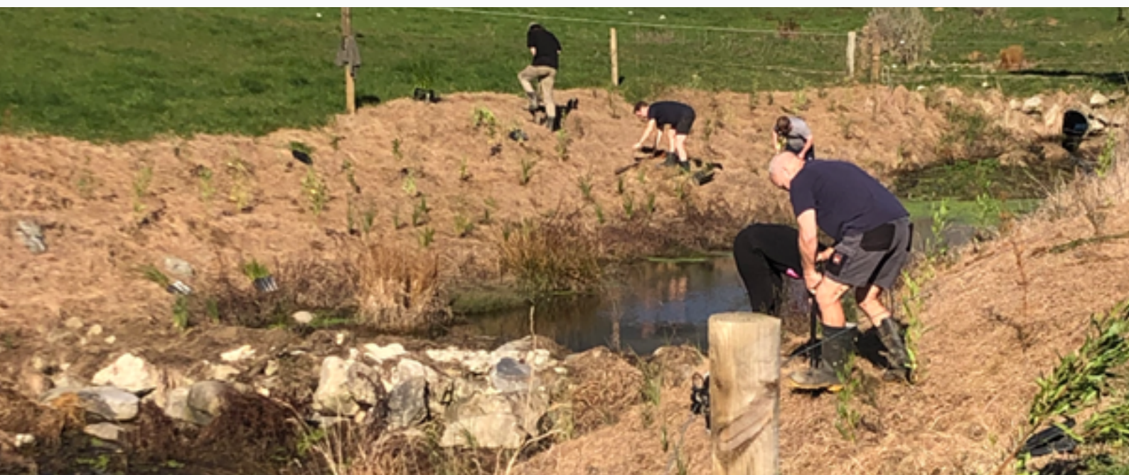
Planting up leaky weir
