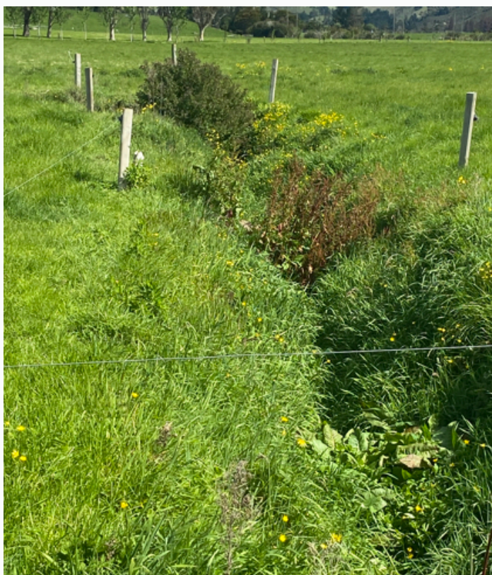
Open drain in Pakahi soils that cattle graze to the edge, removes water quickly but the drain contains filtering vegetation growth
